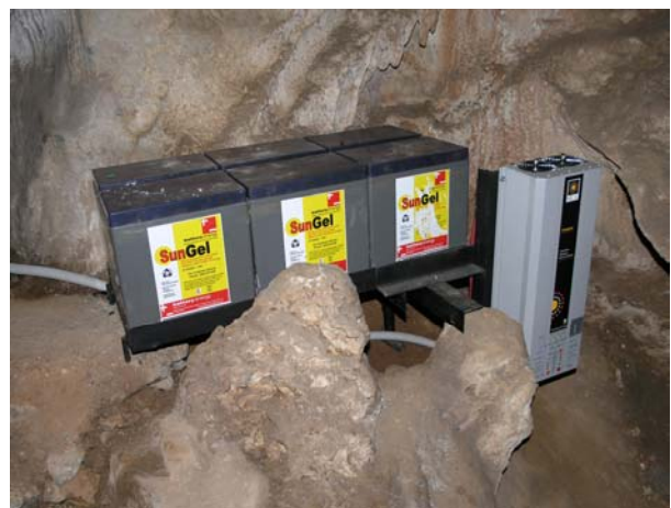
Gel cell batteries and inverter in Lucas Cave. Photo: Russell Commins.
