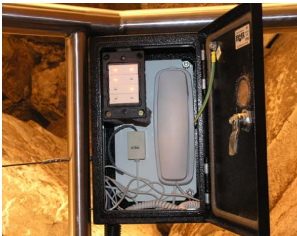
IR Receiver/Backup switching and phone system, Lucas Cave. Photo: Russell Commins.
